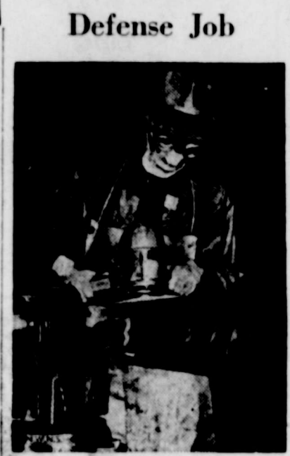
His face protected by an odd-looking mask and goggles, a skilled operator is shown polishing to a high finish a propeller blade in America's largest airplane propeller-manufacturing plant in Caldwell, N. J.
