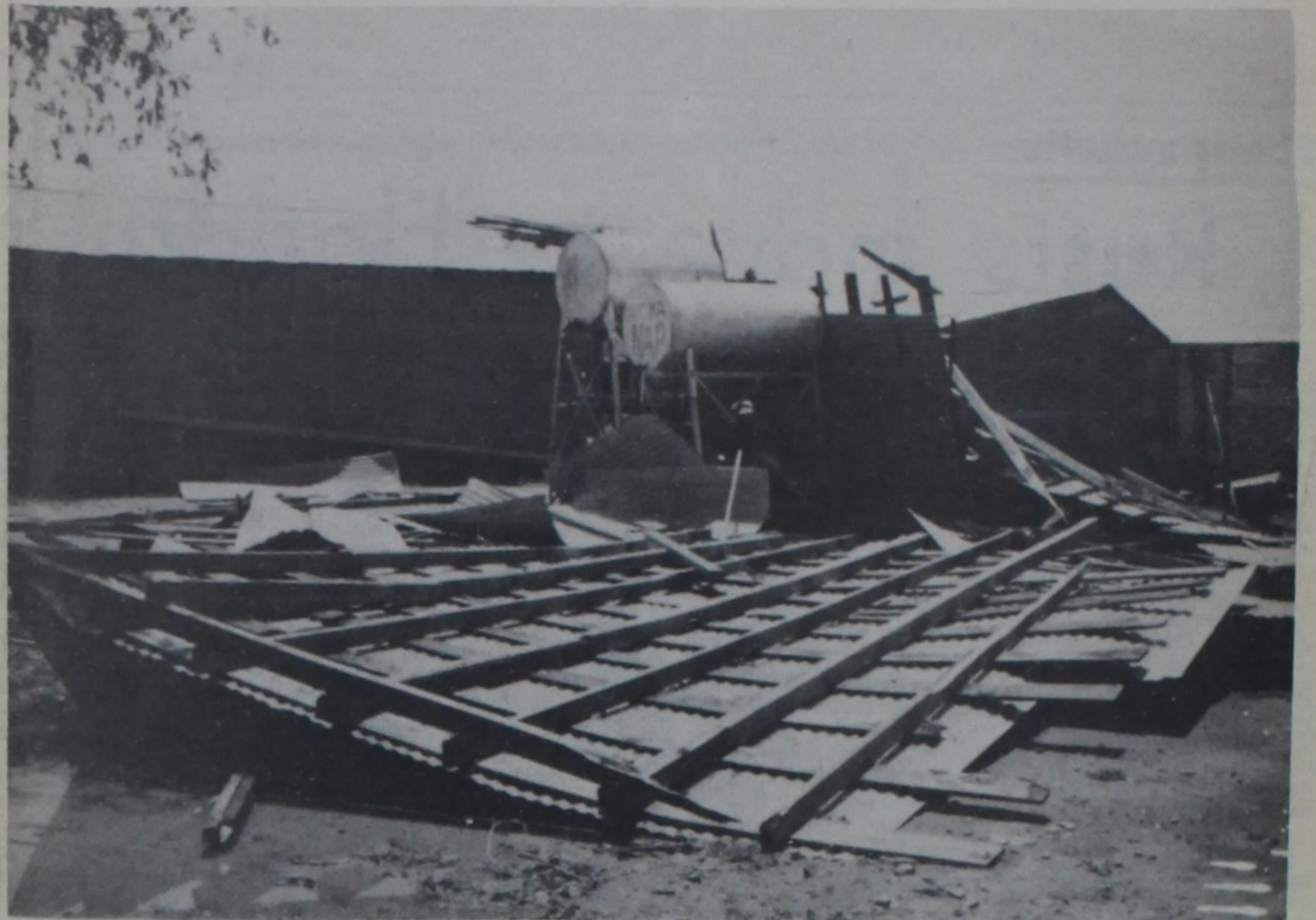
AFTER THE TORNADO, Paul Brooks' barn roof and beams ended up on the opposite (south) side of the main barn. Brooks' son, Thomas Lee, and a hired hand, Feliciano Mata, had just driven their pickups into the barn to escape the
