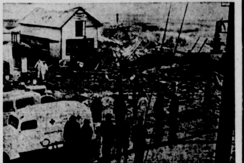
WOODBIDGE, N. J. This scene of desolation met the eye after a terrifying blast leveled the United Railway and Signal Co. plant at Woodbridge, N. J., killing nine persons and injuring 33. Though the plant manufactured torpedo signals for railroads, it was said to be working on a device of "great importance" to the army and navy. Sabotage was suspected.
