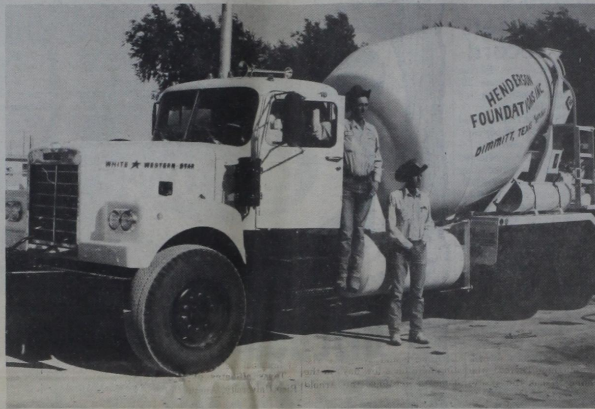
CARL AND STANLEY HENDERSON OF HENDERSON FOUNDATIONS, INC. ... With company's newest concrete-mixer truck
