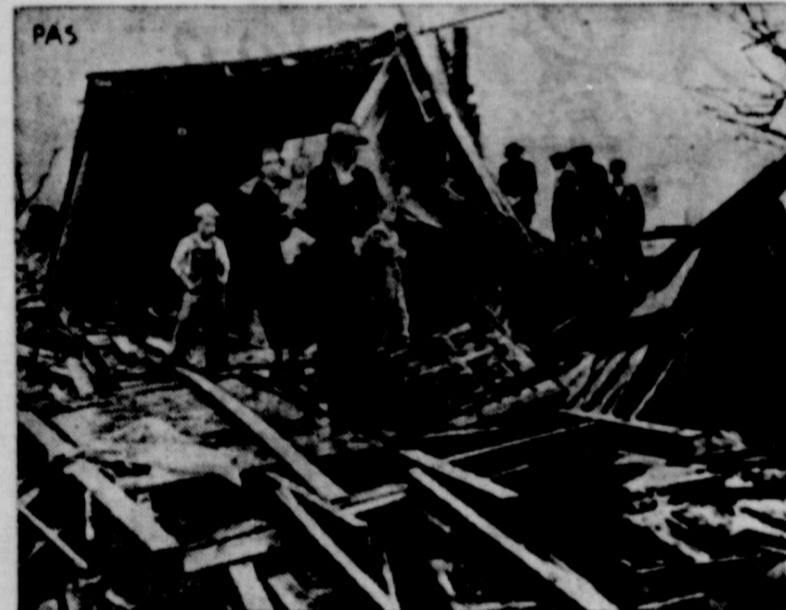
ATLANTA, Ga.—This was all that was left of the five-room home of Mr. and Mrs. Herbie Stancil of near Crabapple, Ga., after a cyclone struck there. Mrs. Stancil was pinned in the wreckage, but escaped with minor lacerations and bruises.
