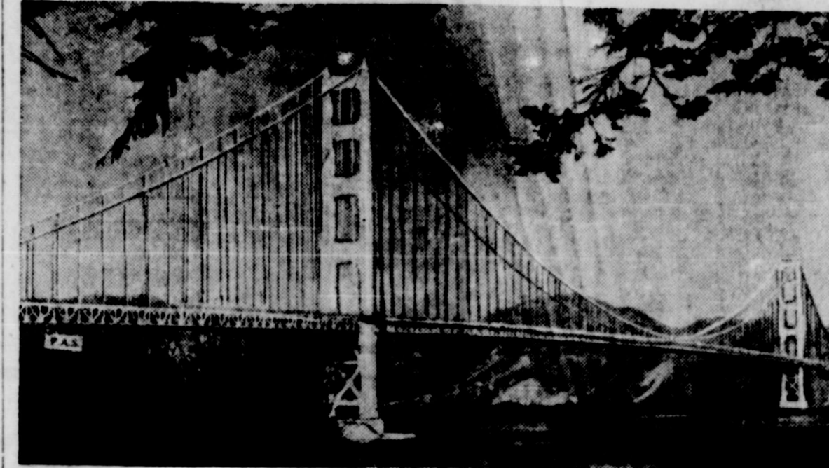
Selected by a jury of leading engineers and architects as the most beautiful bridge built in America during the past year, the Golden Gate Bridge (shown above), across the Golden Gate at San Francisco, Calif., won the highest award, Class A, for monumental bridges. The award is made each year by the American Institute of Steel Construction. Prize awards for smaller bridges were—Class B: Little Hell Gate, Low Level Bridge, New York City—Class C: Chesterfield-Brattleboro Bridge, over Connecticut River—Movable Bridge Class: Marine Parkway Bridge, over Rockaway Inlet, New York City.
