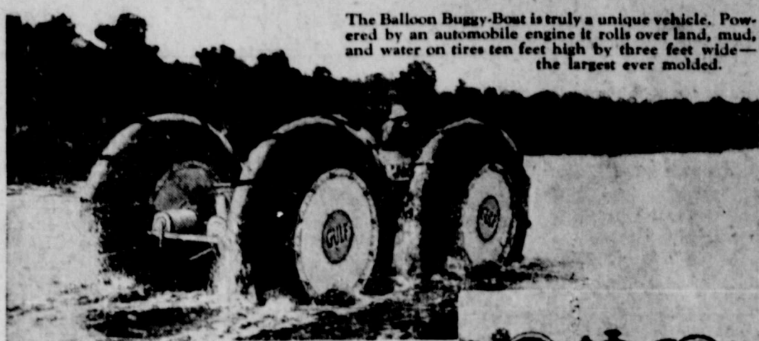
Gulf Oil Corporation engineers call their invention a Marsh Buggy. It is equipped with all the marine requirements for Class I motor boats. Its displacement in water is two feet.
