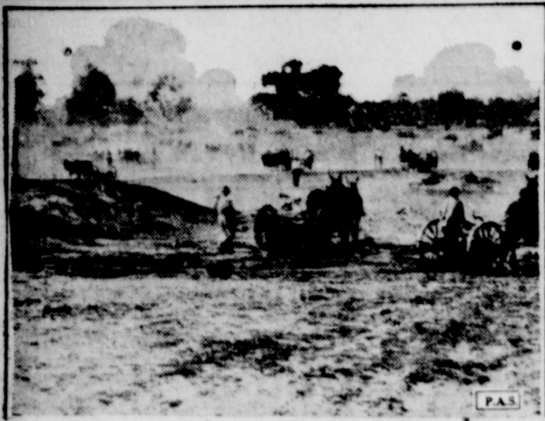
OCALA, Fla. . . . Hundreds of mule-drawn scrapers are biting into Florida soil, digging the path which will be a sea-going ship canal across the state, joining the Gulf of Mexico with the Atlantic Ocean and thus taking coastwise ships out of the hurricane zone around the keys.
