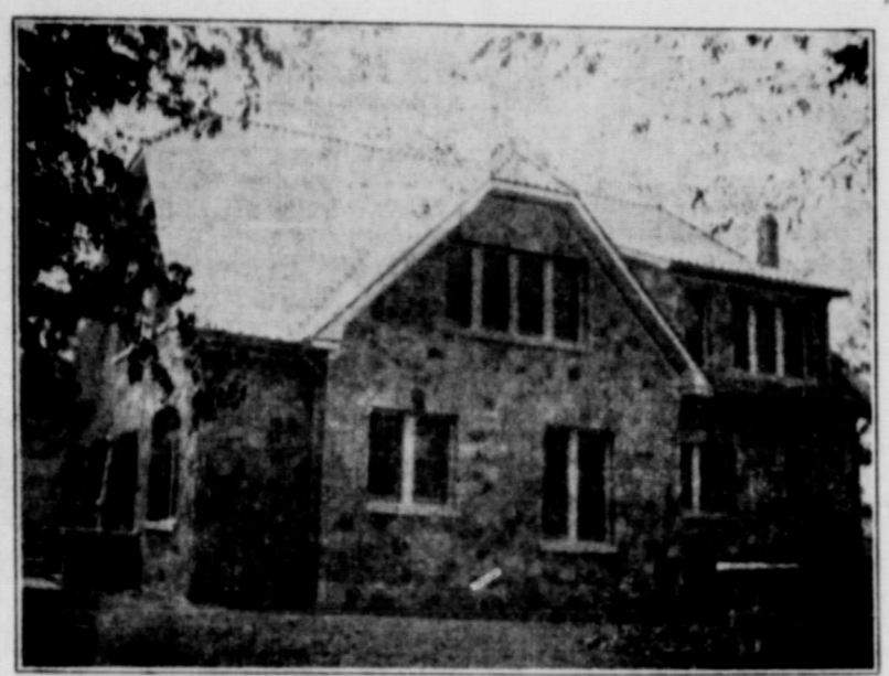
View Taken From North Side of House
