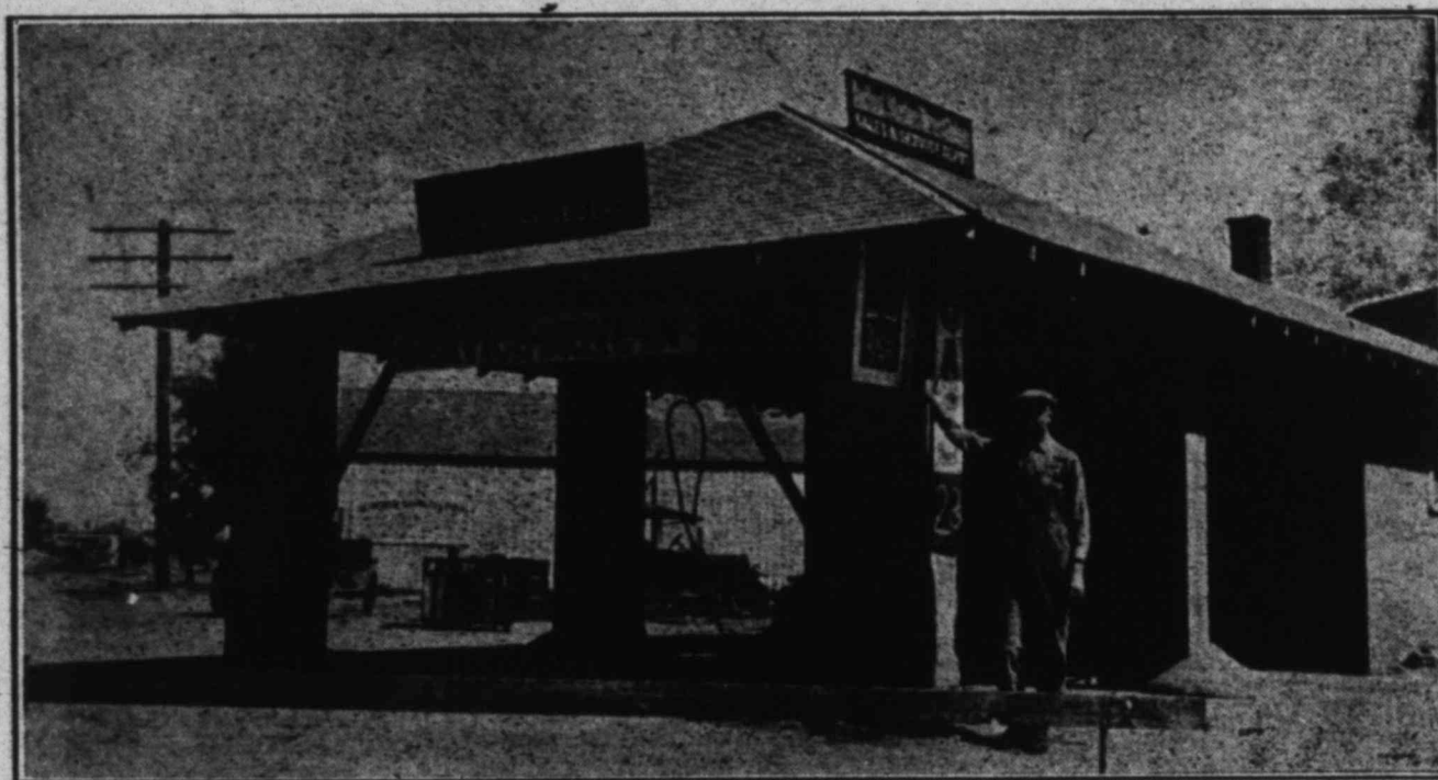
G. W. JOHNSON FILLING STATION
