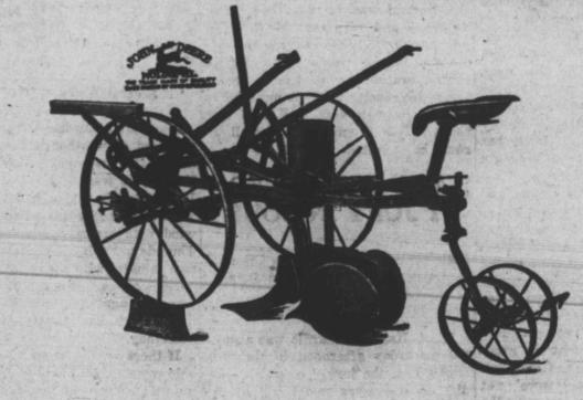
With leveling lever on each front wheel and foot lever lifting device.
