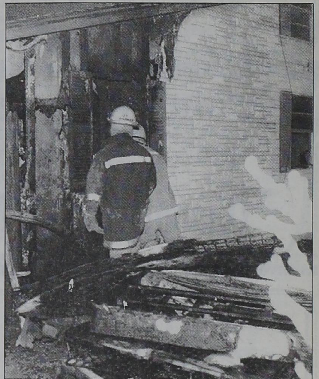
VOLUNTEER FIREFIGHTERS look into the window of a house that was damaged by fire Friday night in Dimmitt. No one was injured in the fire, which was at the home of the Johnny Lugo family on South Broadway. The fire started in the back bedroom and several flaming mattresses were thrown out this window during the effort to extinguish the fire.
