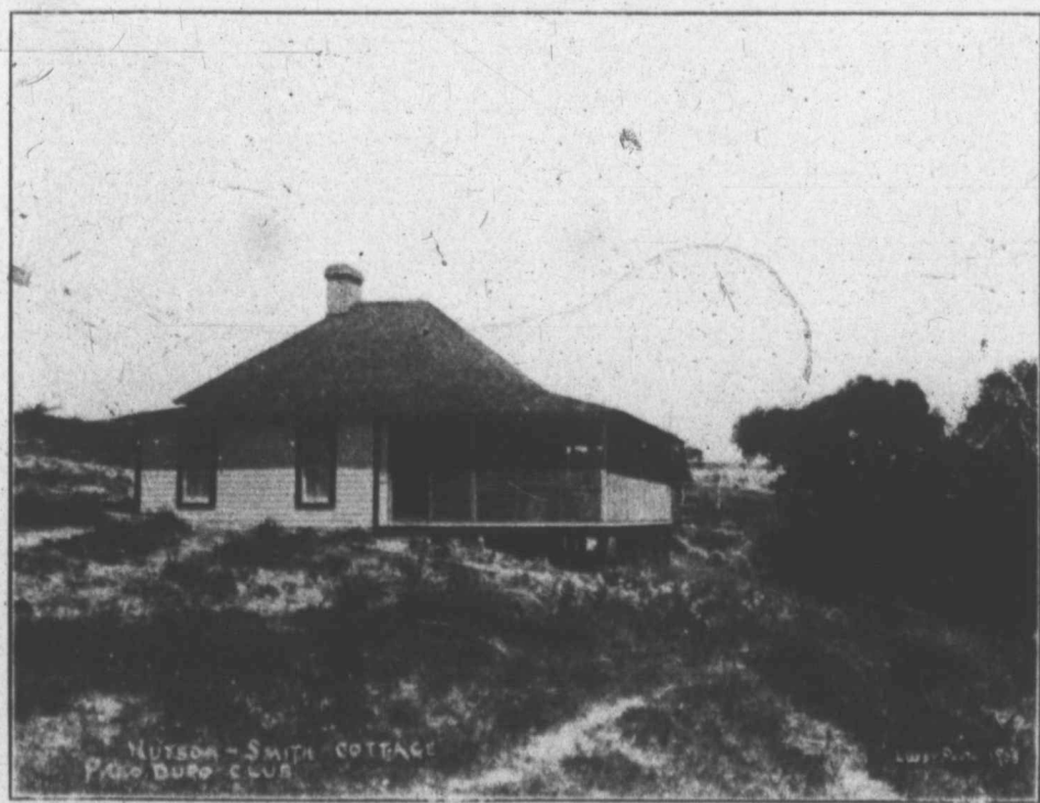
Members of the Palo Duro club often spend weeks at their club houses on the club grounds. The house here shown is that of John Hutson, Heberd Smith and Clark Smith, which will give an idea of the cottages which the members build there for their own use. Large general cottages are maintained for the members who do not have the private buildings. The deep declivities, the cool, inviting nooks and shady places, the splendid fishing facilities and the elegant cottages and club houses make the club grounds a well chosen place of recreation and rest for members.
