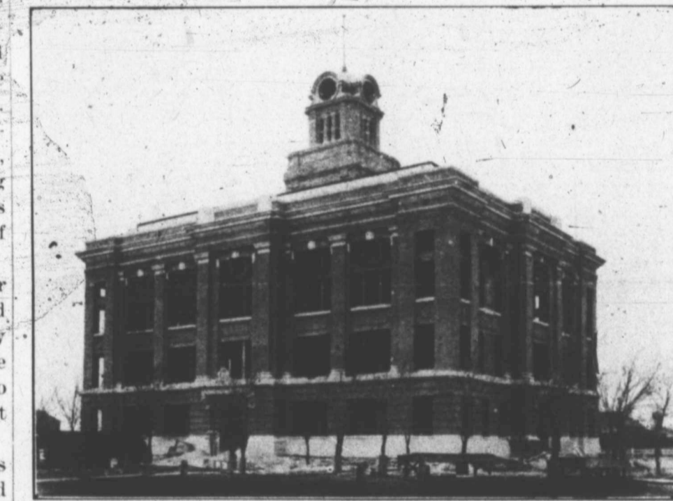
Herewith we present a picture of the new court house which is now rapidly nearing completion. It is a handsome three-story brick building trimmed in carthage marble and terra cotta and is the most conveniently arranged court house in the entire west. The building exclusive of the tower clock and the inside furnishings is to cost $53,500 when completed and the work is being done by Messrs. Gilcoat & Skinner, contractors, of this city. The plans for this handsome edifice were made by the R. G. Kirsch Architectural Company of St. Louis, Mo., the contract for the plans having been awarded to them after spirited contests. There is not a handsomer nor a better constructed building of the kind in Texas—and the people of Randall county are more than pleased with it.
