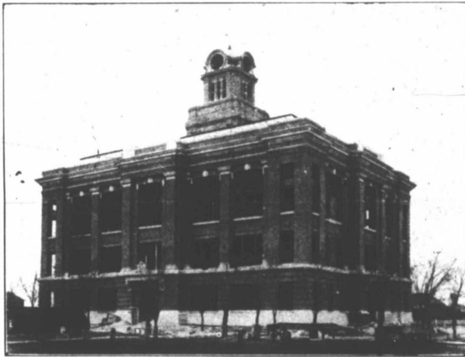
Herewith we present a picture of the new court house which is now rapidly nearing completion. It is a handsome three-story brick building trimmed in carriage marble and terra cotta and is the most conveniently arranged court house in the entire west. The building exclusive of the tower clock and the inside furnishings is to cost $53,500 when completed, and the work is being done by Messrs. Gleason & Skinner, contractors, of this city. The plans for this handsome edifice were made by the R. G. Kiesch Architectural Company, of St. Louis, Mo.; the contract for the plans having been awarded to them after spirited contests. There is not a handsomer nor a better constructed building of the kind in Texas, and the people of Randall county are more than pleased with it.
