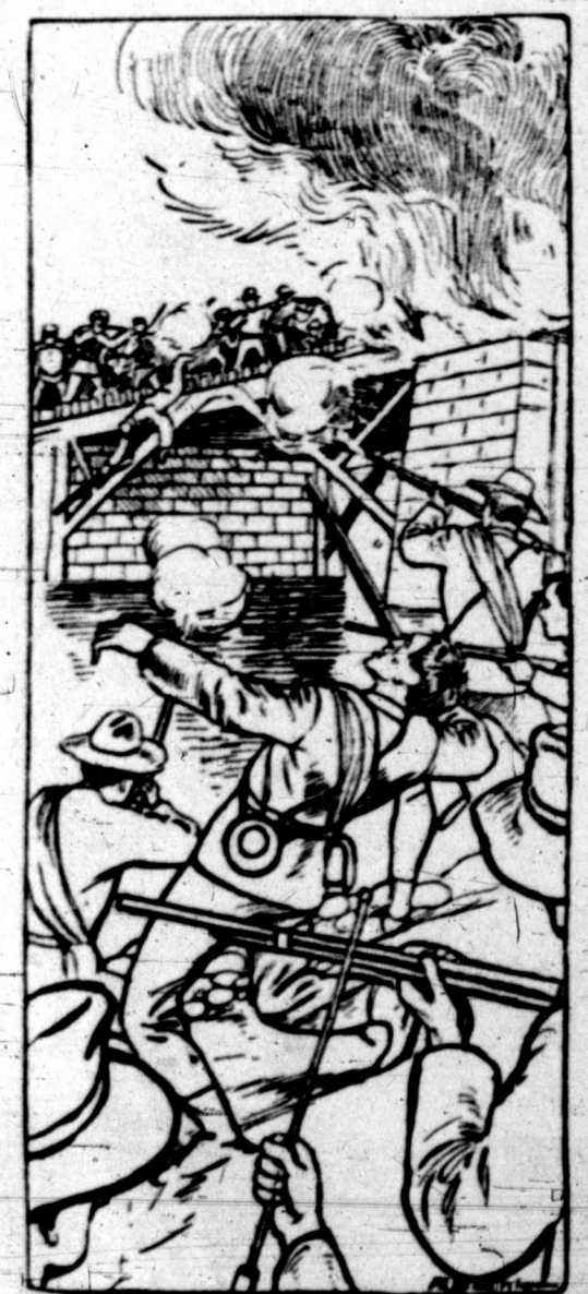
BARLOW'S MEN CROSSING APPOMATTOX BRIDGE
