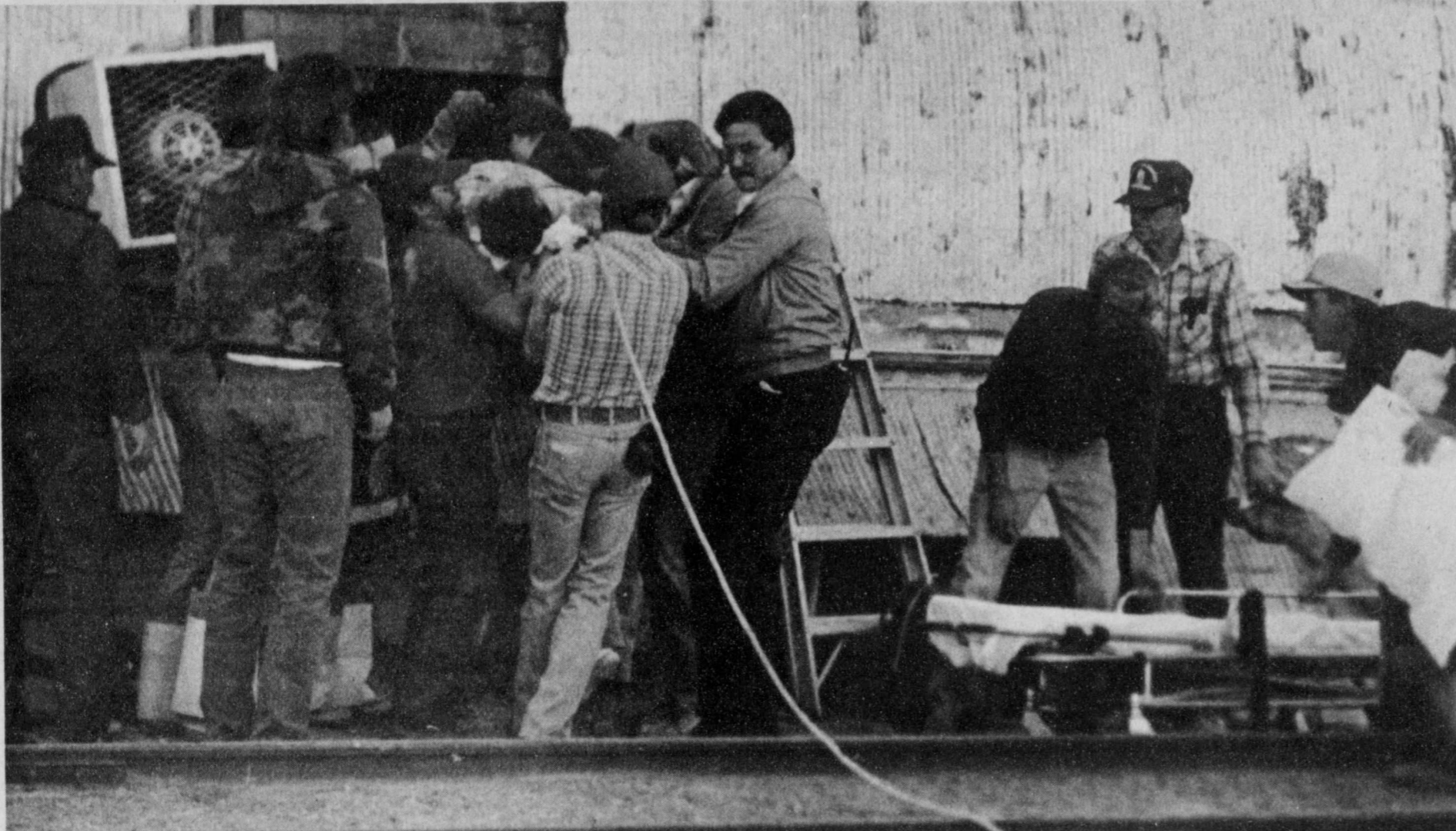
RECOVERY COMPLETE — Members of Lockney and Floydada fire departments, two peace officers and others ease Gene Watts of Floydada through a hole in the side of a Muncy Elevator structure after he suffered a fall — believed to have been
