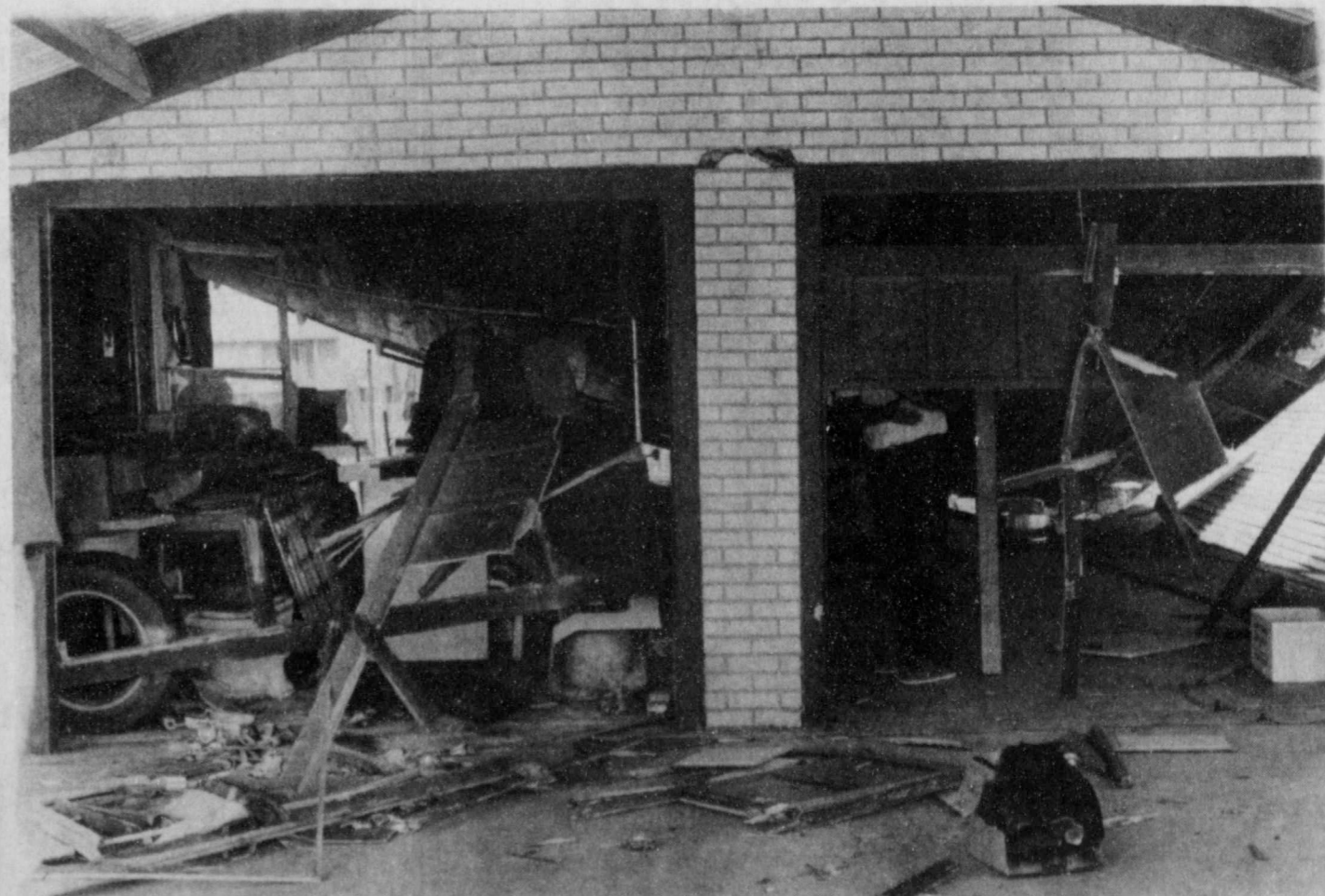
HOME EXPLODES — As of press time no final determination had been made as to the cause of the explosion that destroyed the garage of the Homer Ragland home last Monday night. Not only did the explosion destroy the garage but it broke
