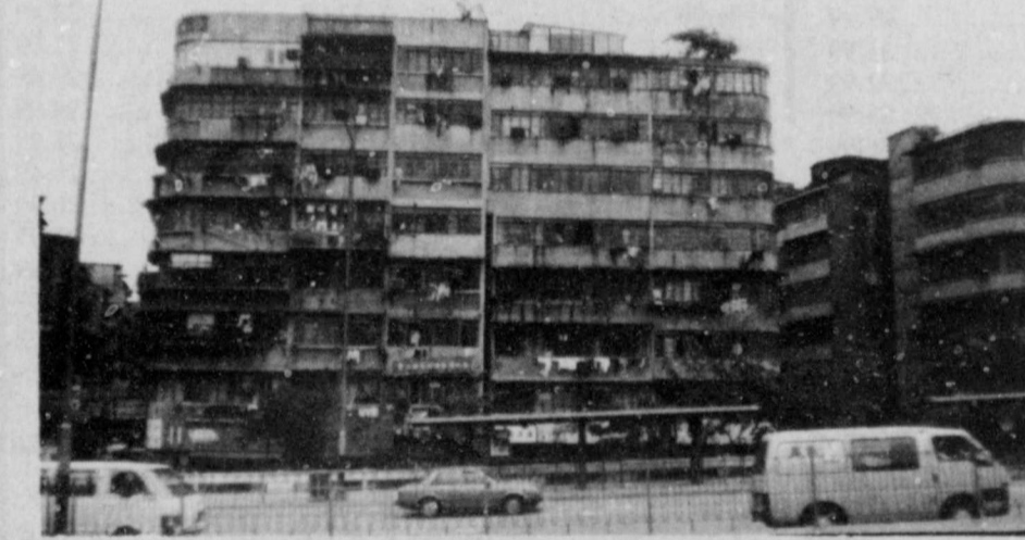
MOST OF THE APARTMENT BUILDINGS we saw were older, and all had laundry hanging out the windows or strewn across a balcony. Hong Kong is not an especially pretty city; their main trade is definitely tourism.
