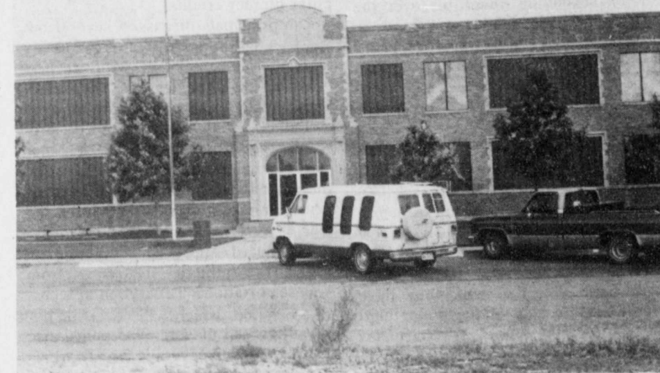
FOR THOSE WHO HAVE NOT been by the High School and Junior High buildings recently you may not have noticed the improved look. The building have been chemically cleaned, all the cracks have been repaired, the missing tiles around the top of the building have been replaced, and the buildings have been sealed.
