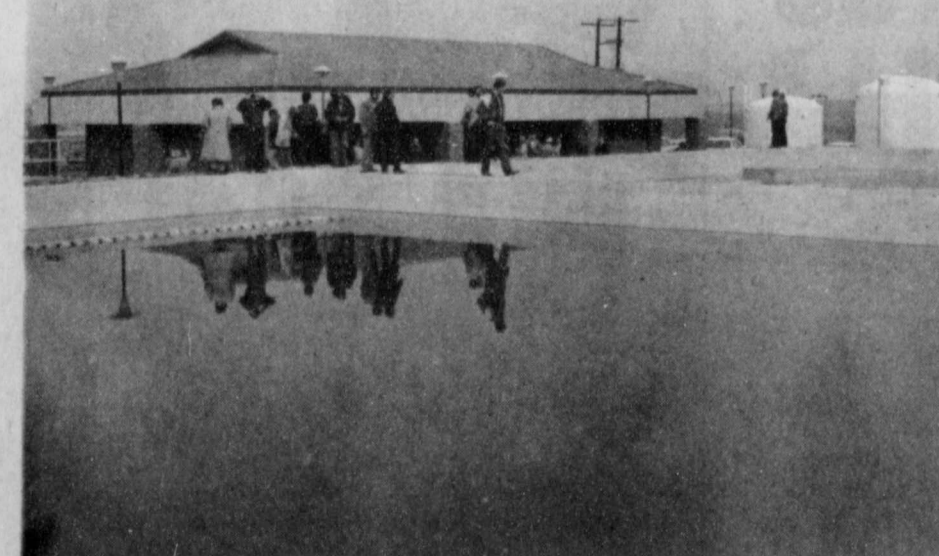
AFTER THE WATER from the Mackenzie project is mixed with alum and chlorine it is sent to the filtering basins shown here.
