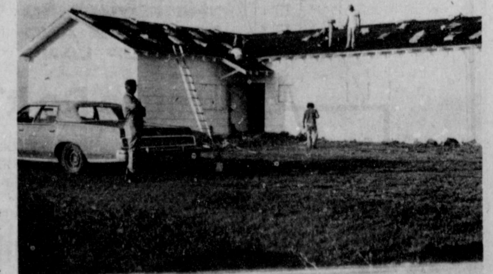
GEORGE ALBERT watches as a crew starts to reshingle the Evans Baptist Church on Locust Street. Further remodeling is planned for the future to the inside of the building.
