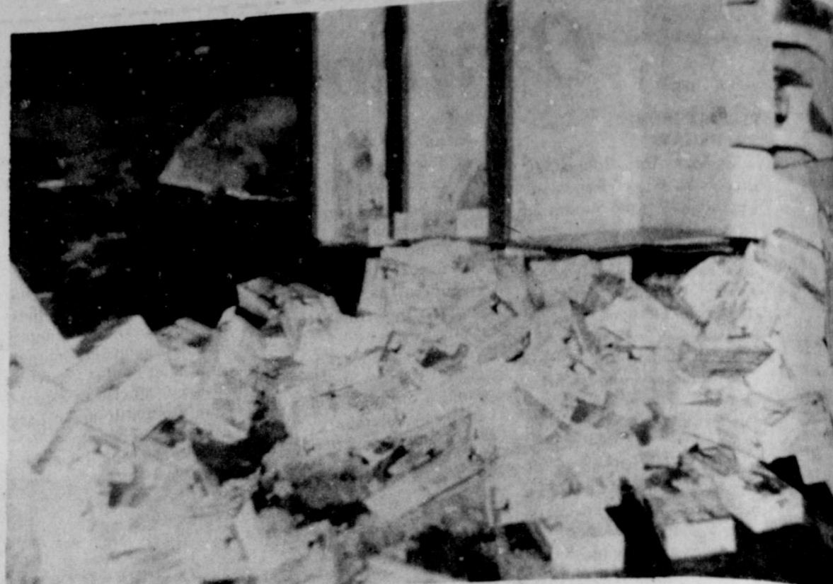
There was extensive smoke and water damage in the fire at Keeter's Grocery.
