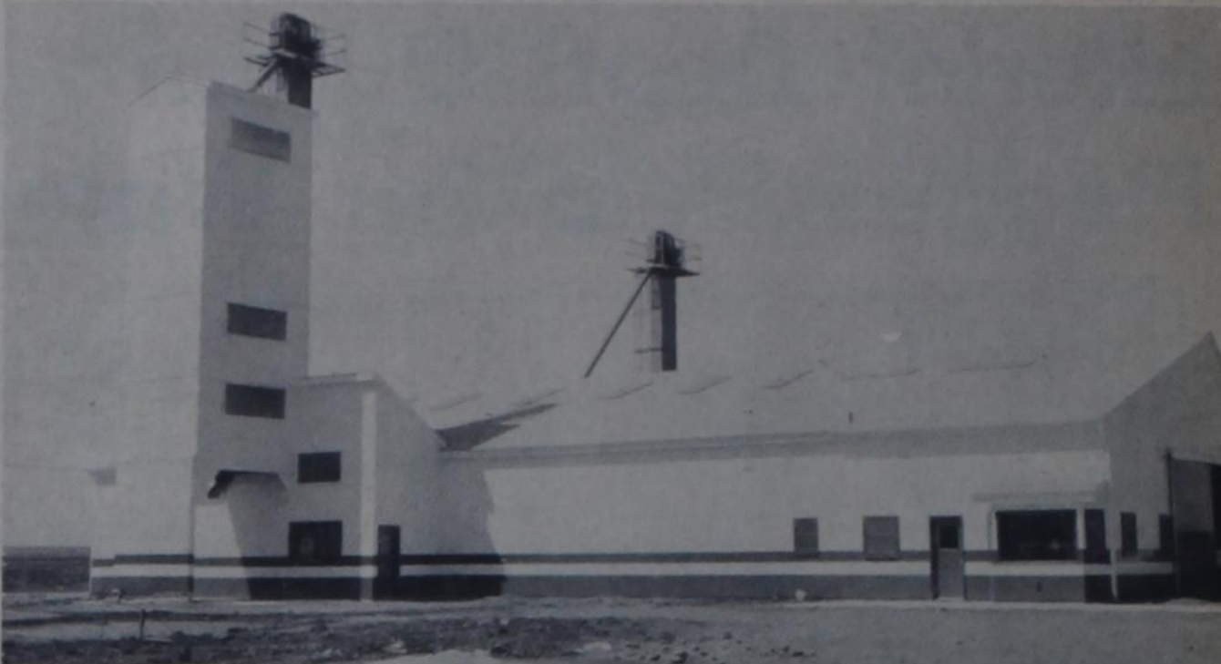
THE FINISHED PLANT being built here by American Cyanamid Co. will look like this. At left is a cluster of blending bins that will mix dry fertilizers over a loading dock.
