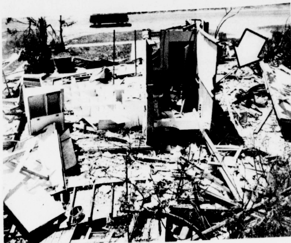
A SINGLE WALL remained at the Gene Ehler residence following a May 11, 1970, tornado which ravaged Lubbock.
