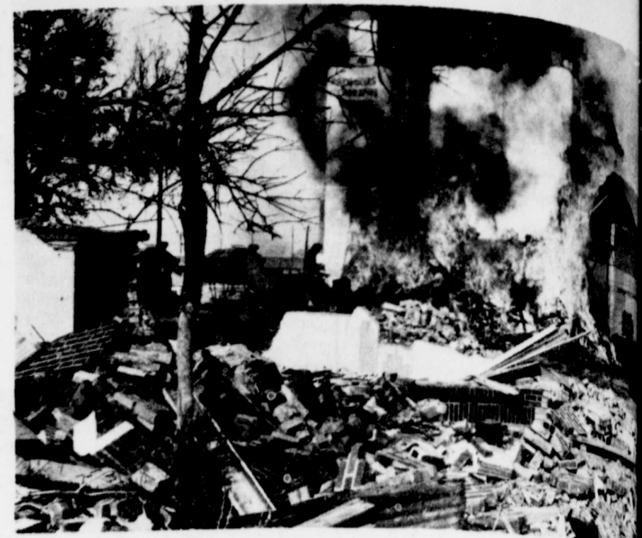
ELEVATOR BURNING?? At first glance one would think so but debris left after the structure of the old Willson and Son Lumber was destroyed. The building was one of the few remaining early day businesses in Floydada erected in 1920.
