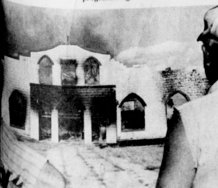
... DEMOLITION of the old city auditorium continued Wednesday morning. (Staff Photos)
