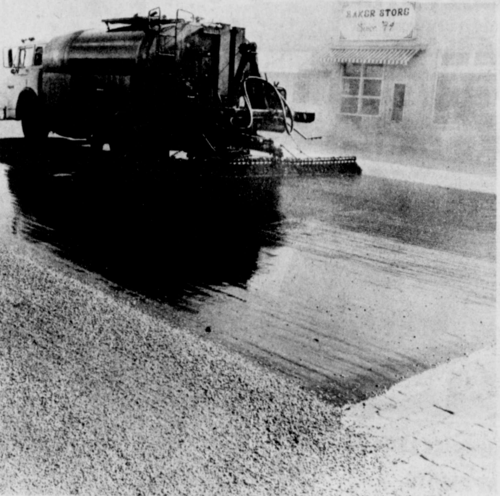
MAIN STREET (and other streets in Lockney) got "tarred and gravelled" Thursday. The city of Lockney seal costs several blocks of city streets each year. (Staff Photo)
