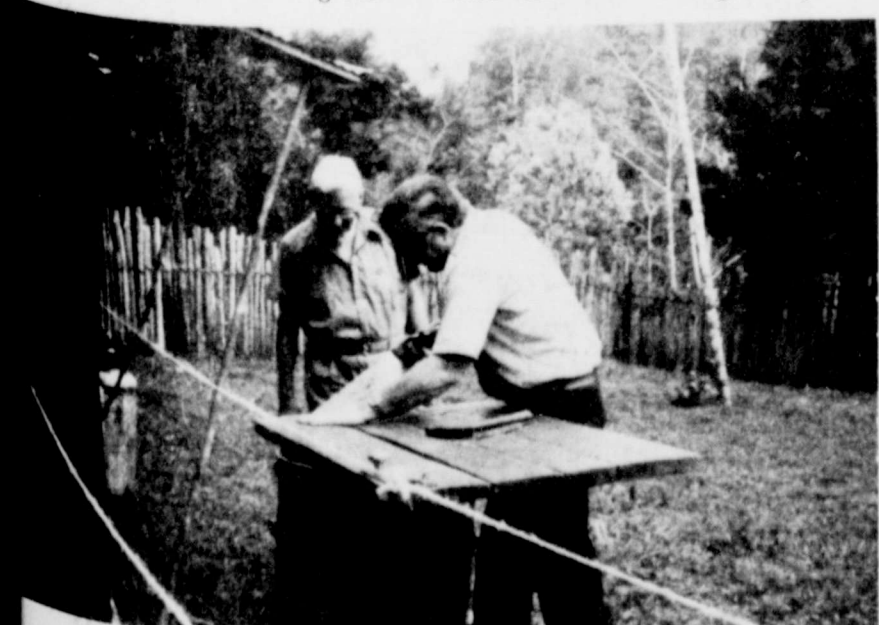
JACK MCINTOSH AND LOUIS LLOYD on a building project.
