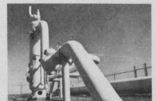
So was natural gas.
