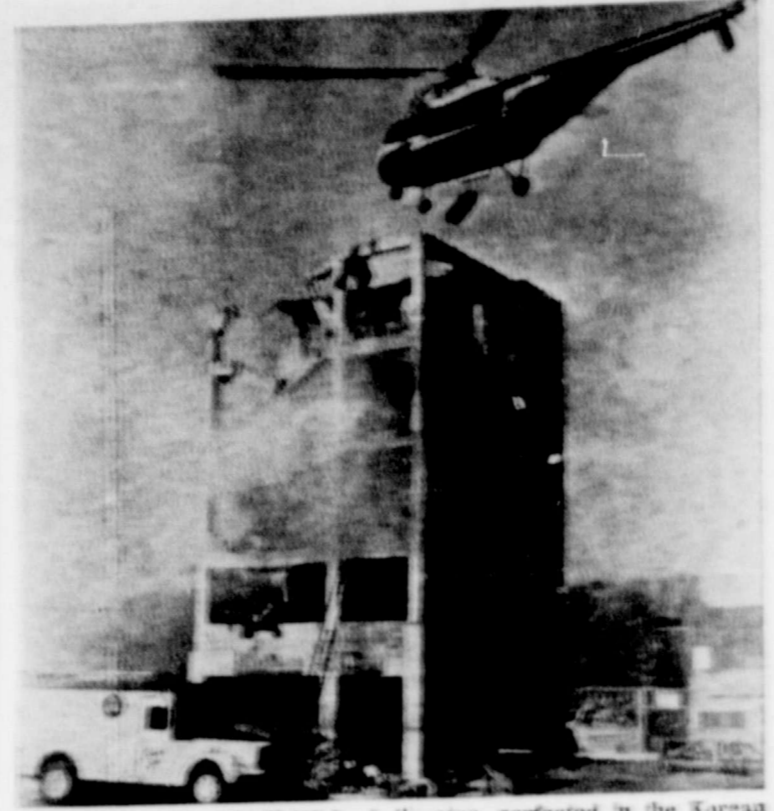
CASUALTY EVACUATION by helicopter, perfected in the Korean War, is demonstrated at the Federal Civil Defense Administration's up-to-date rescue school at Olney, Md. Here a street of carefully engineered "bombed out" buildings confront rescue course students with a variety of situations, including rescue from actually flaming structures of persons made to as "victims." (Sam Photo)
