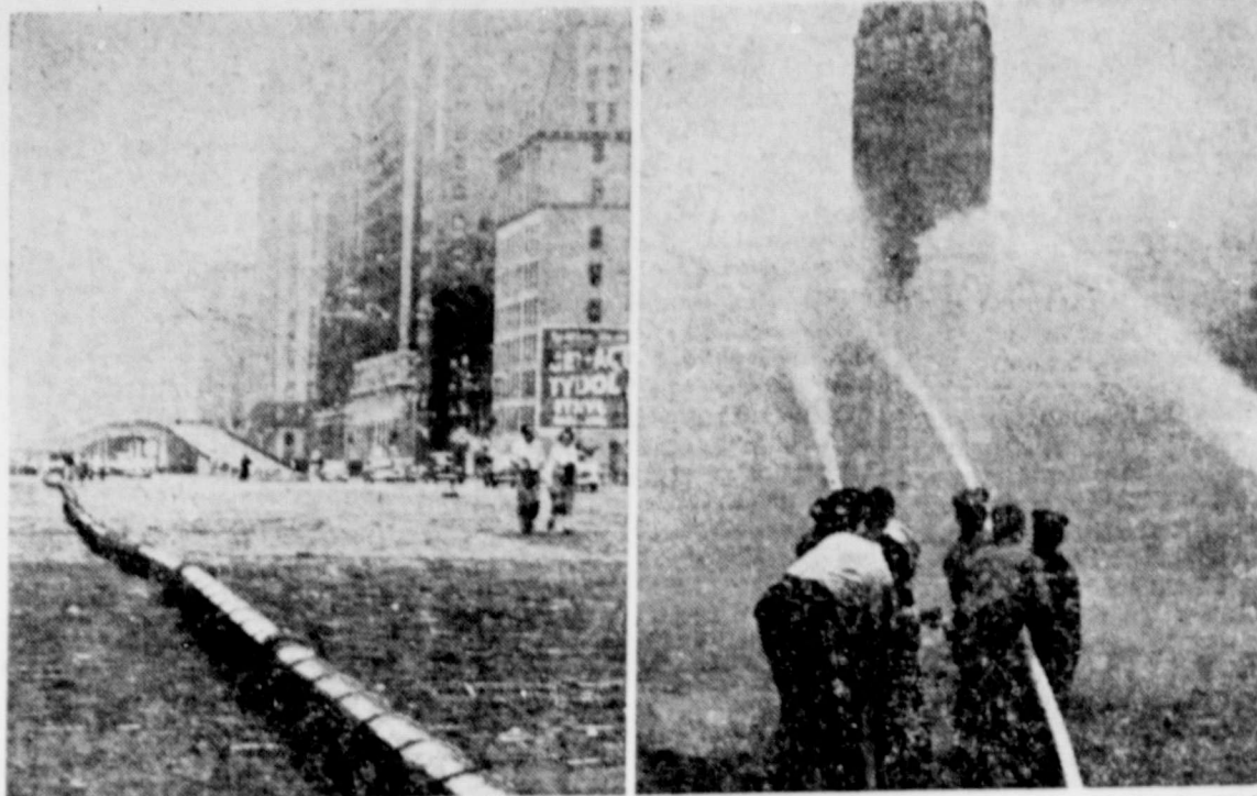
DEMONSTRATION OF PIPE in New York City which can be laid quickly over rough terrain to carry water for fire fighting, city water supply or to pump out flooded areas. This flexible-coupled pipe is stored by the Federal Civil Defense Administration in warehouses throughout the nation for use in emergencies. New couplings allow pipe to be laid without leveling it.
