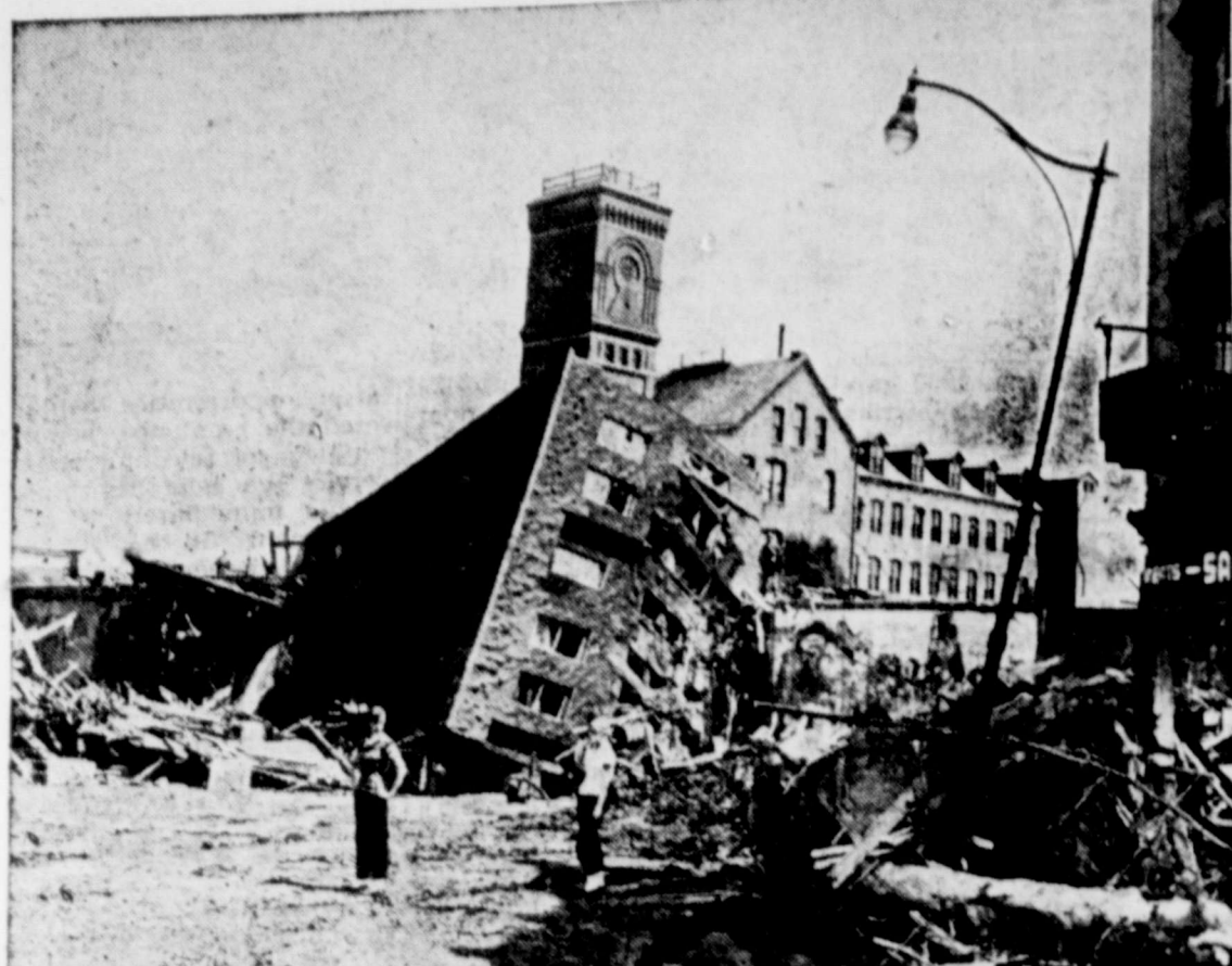
CRUSHED AND BROKEN, this 16-family apartment house in Waterbury, Conn., was left high and dry after the rampaging Naugatuck River receded August 21. This was a sample of devastation in the flood which, according to the Red Cross, destroyed 1,326 houses and badly damaged 4,808.
