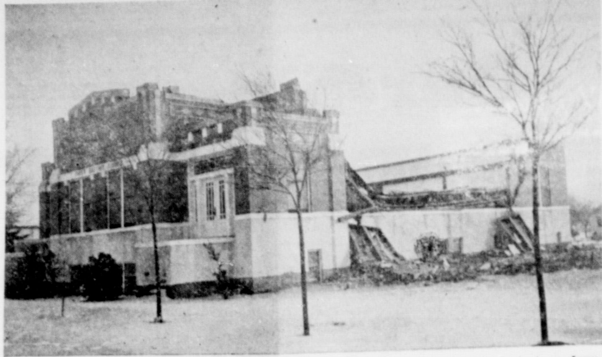
WRECKED — Pictured here is the wrecked building of the Lockney Baptist Church after the roof had caved in from a heavy load of sleet on January 12, 1949.
