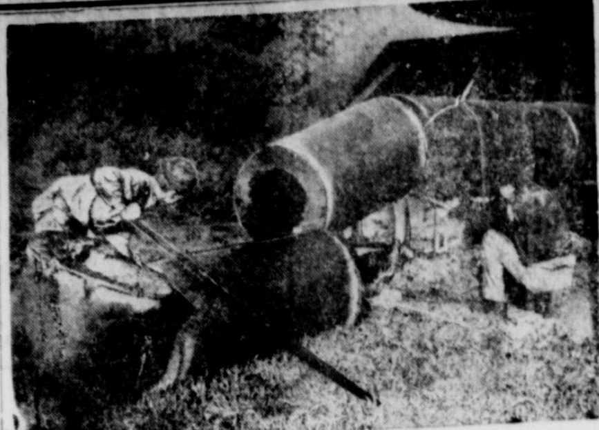
OBSELETE DEFENSE . . . Huge coastal defense guns became obsolete as the bow and arrow with the development of the airplane. This big 16-incher at Fort Fuston, built to defend San Francisco bay, is in the process of being cut up for scrap. The gun is 63 feet long and weighs approximately 370 tons. The barrel is being cut into five sections weighing about 23 tons each.
