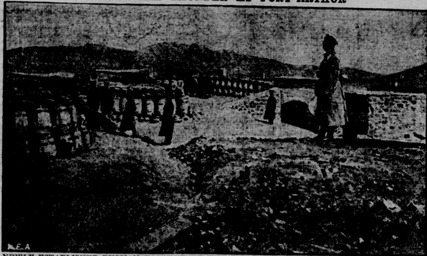
A NEWLY ESTABLISHED RUSSIAN BATTERY AT PORT ARTHUR ABOUT TO OPEN FIRE ON THE JAPANESE. THE WORKS ABOUT THE GUNS ARE MADE UP OF BARRELS FILLED WITH SAND AND COVERED WITH LAYERS OF SAND BAGS.
