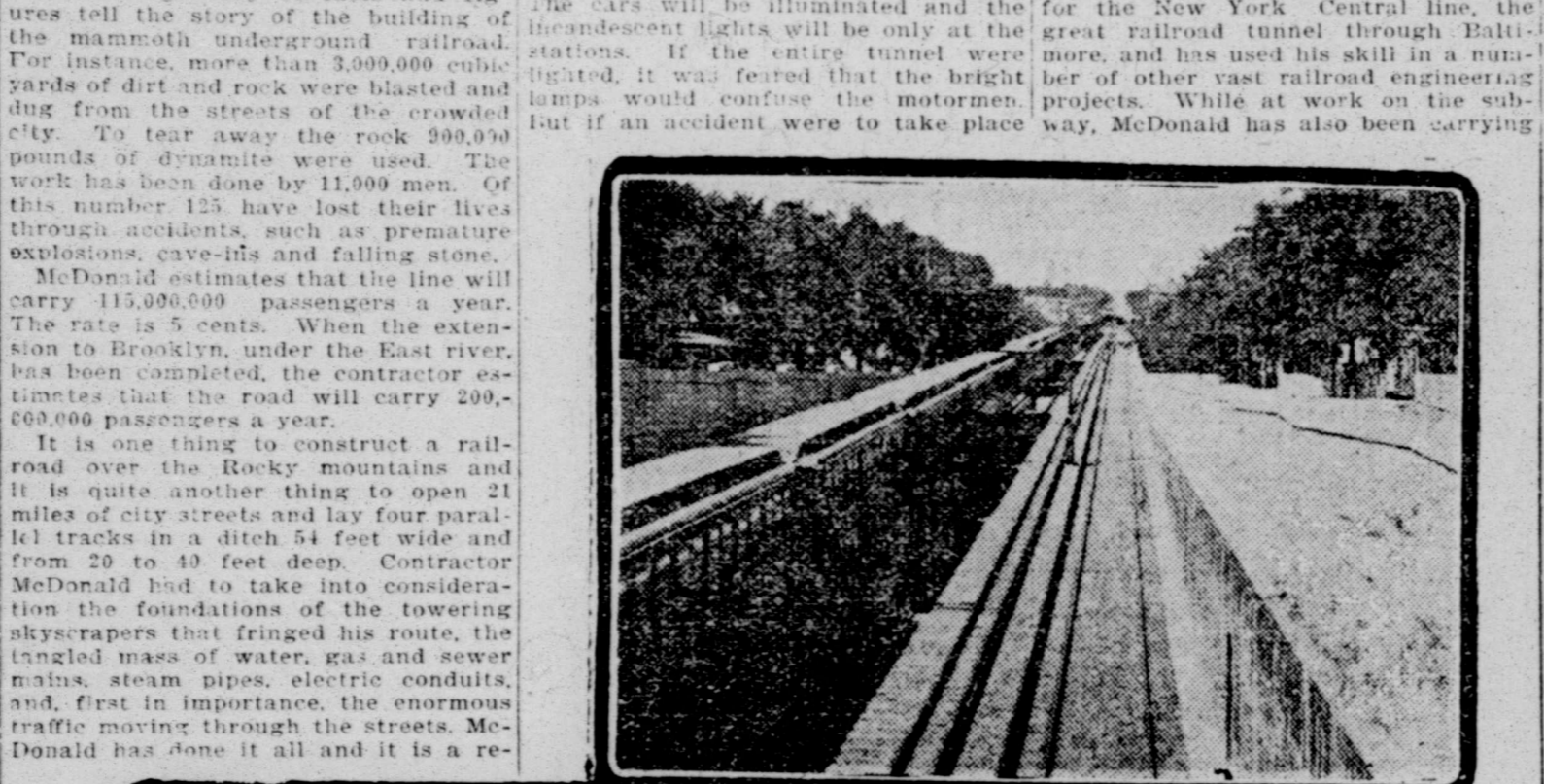
TRAINS EMERGING FROM TUNNEL ONTO VIADUCT AT ONE HUNDRED AND TWENTY-SECOND STREET.
