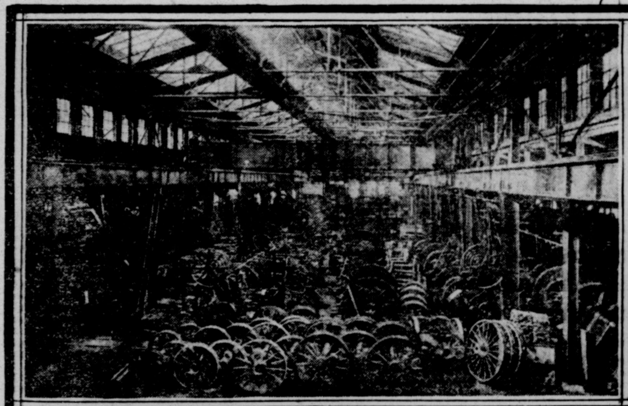
THE WHEEL LATHE SHOP
