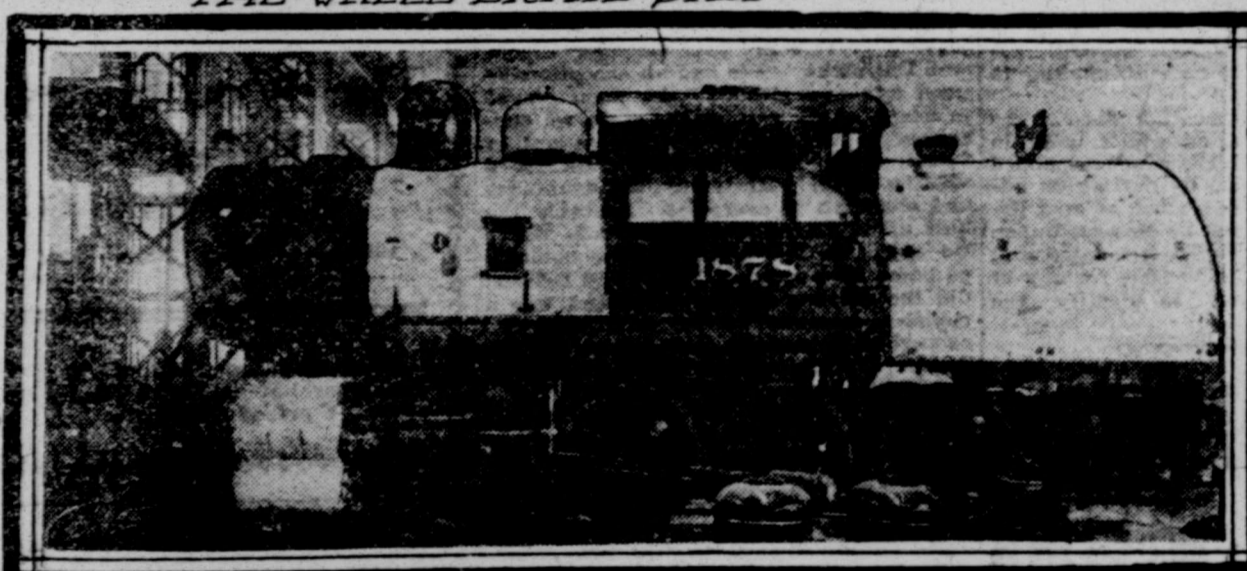
BOILER READY FOR JACKET
