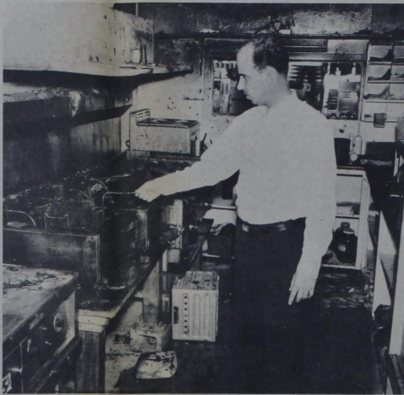
WHERE IT STARTED — Jerry Summers, owner and operator of the Arrowhead Drive-In, shows where Saturday morning's fire apparently started—in this deep "fry-olator," which was left simmering when
