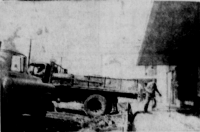
AUSTIN STREET SPRUCE-UP - (Upper) View of free parking lot for customers of Quality Food Mart, corner Main and Austin Sts. (Lower) Preparation for a new and wider sidewalk at Southwest Machine and Engineering Co., 212 North Austin St.
