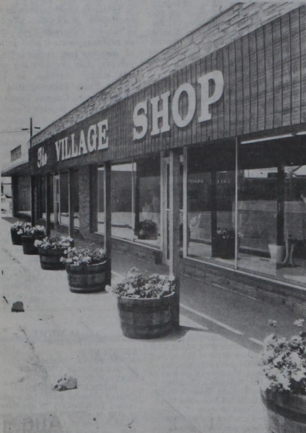
COMMERCIAL BEAUTY SPOT for the first half of June is the Village Shop at 204 West Bedford. The store was chosen because of the decorative planter barrels and work that has been done to improve the outer appearance of the building. Commercial and residential beauty spot nominations may be submitted to the Dimmitt Chamber of Commerce office at 115 West Bedford, or by calling 647-2524.
