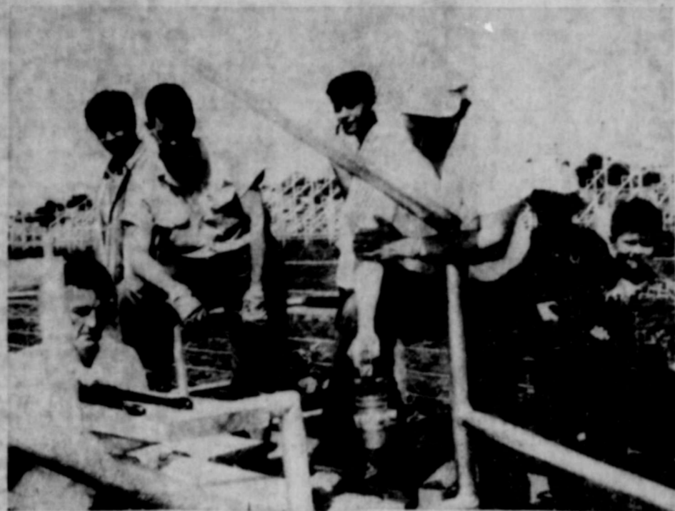
INSTALLING SEATS — The Ranger Jaycee Club is busy these days making necessary repairs and preparations for their big rodeo program July 8-9 as the above picture will show. The work party was repairing the stands when the picture was made. Shown, left to right, are Doyle Gentry, Ernest Nunez, Fred Bennett, Beto Jimenez, Don Yarborough, Donald Yarborough and little Richard Fletcher. (Photo courtesy Capp's Studio.)
