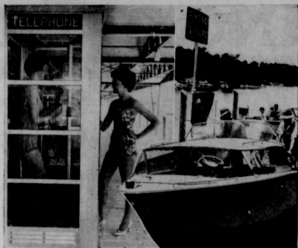
WATER PHONE —This floating telephone at Eisenhower State Park Mariana on Lake Texoma near Denison enables users to call anywhere in the country without leaving their boats. This drive-in public telephone for boats is the first installation of its kind in the nation, according to a Southwestern Bell Telephone Company spokesman. The telephone is affixed to a dock floating in water about 100 feet deep. Using the telephone is Mary Sue Huff. Barbara Pierce is at the steering wheel. Both are Denison telephone employees.
