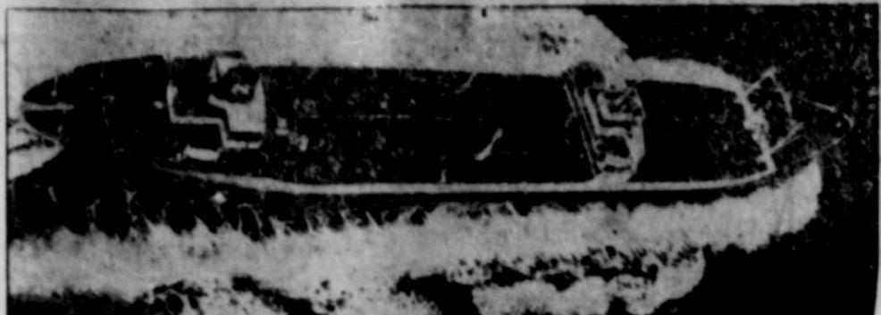
LARGEST TANKER SHAKES DOWN—Whipping the water to a froth the tanker "World Glory," largest cargo ship ever built in the Western Hemisphere, speeds through shake-down tests off the coast of Maine. Built at the Quincy, Mass., yards of Bethlehem Steel, the huge craft is 736 feet, 3 1/4 inches in over-all length, has a breadth of 102 feet, depth of 90 feet and a draft of 37 feet, 6 1/4 inches. She is designed to cruise at 16 knots and has capacity for over 16,000,000 barrels of oil.
