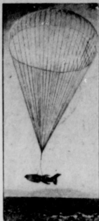
'CHUTE, THE WORKS—Its test run completed, a Ryan "Firebee" guided missile is lowered to the desert in New Mexico on its own 50-foot parachute. The parachute, which may be operated either by remote control or automatically, saves the expensive, 600-mile-per-hour device for further tests.
