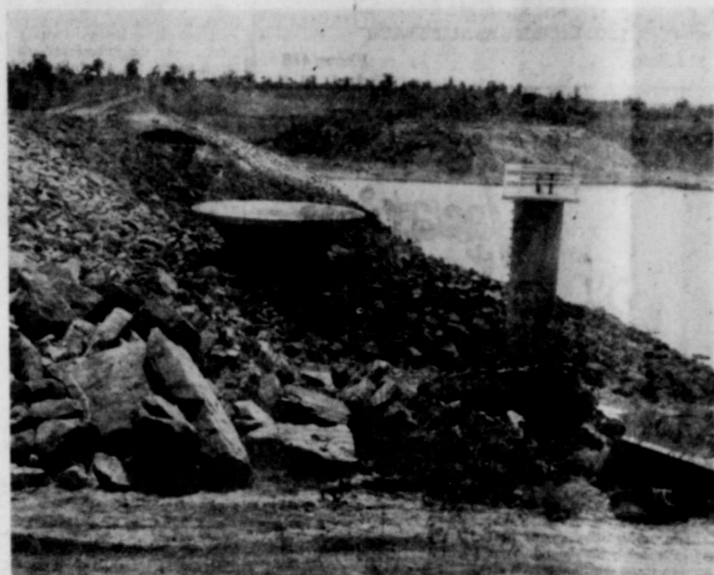
BACKING UP WATER—The new Ranger-Eastland lake on the Leon River has already begun forming back of the huge dam built by the Eastland County Water Supply District. The picture above was taken facing south. The coin shaped cement work at left is the overflow valve and the tower at right is the safety valve. The gap which is at present being filled can be seen in the center of the picture. (Times Staff Photo).
