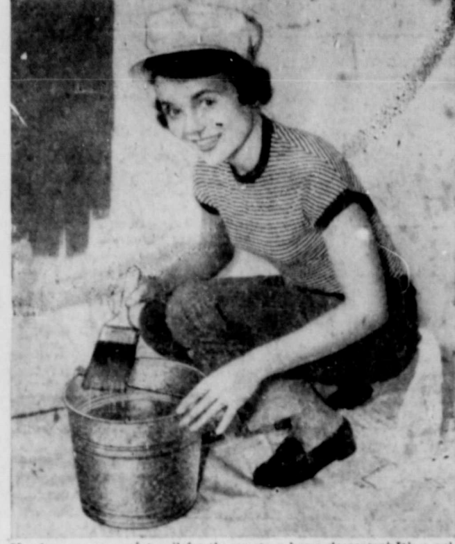
Here's a no-mess paint pail for the amateur home decorator! It's a galvanized steel pail with a wire stretched across the top and fastened to the pail's handle attachments. The wire, instead of the pail's edge, is used to remove excess paint from the brush, thus letting the paint fall back into the pail.
