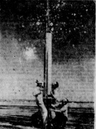
ALL-AMERICAN ROCKET-THE WAC CORPORAL-is smaller than the 14-15 ton German V-2. Developed in 1945, the experimental, liquid-fuel, high altitude rocket weighs 655 pounds with a fuil fuel load and attains a top speed of approximately 2,800 miles an hour.
