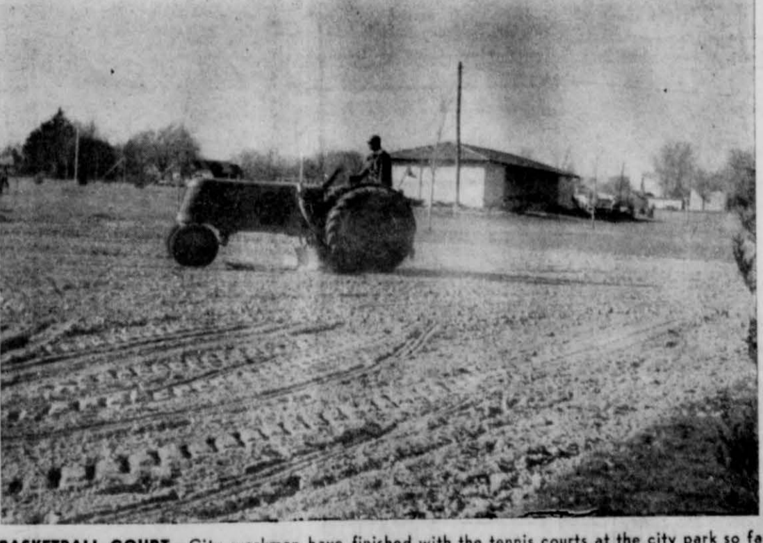
BASKETBALL COURT—City workmen have finished with the tennis courts at the city park so far as the base is concerned and are engaged in finishing up the basketball and volleyball courts above. They will be topped with a cold asphalt mix and will be ready for use in early summer or late spring.
