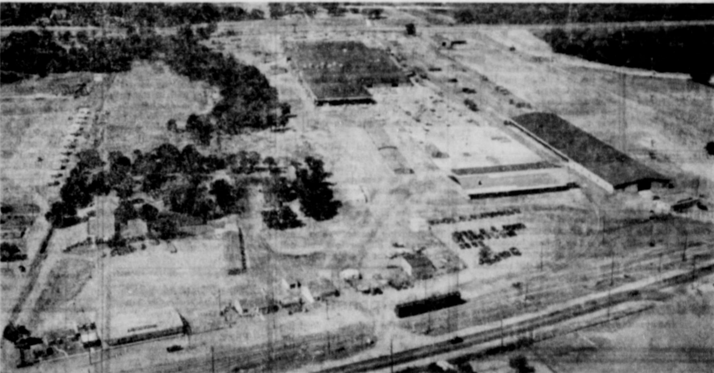
42-Acre Plant Site of Texas Housing Company, 9001-03 Denton Drive, Dallas, Texas, with six acres under roof, equipped with modern wood-working machinery, and nine acres concrete loading area served by double railroad switching and loading tracks.
