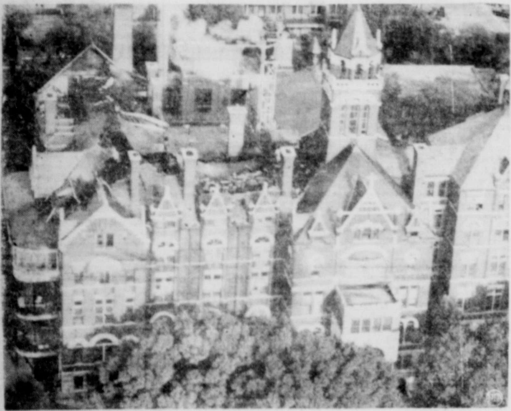
ST. PAUL HOSPITAL WING DESTROYED—More than 250 patients in the St. Paul Hospital in Dallas were evacuated by Nuns and Nurses without loss of life after a midnight blaze razed the west wing nurses dormitory (upper left) of the hospital. (NEA Telephoto).
