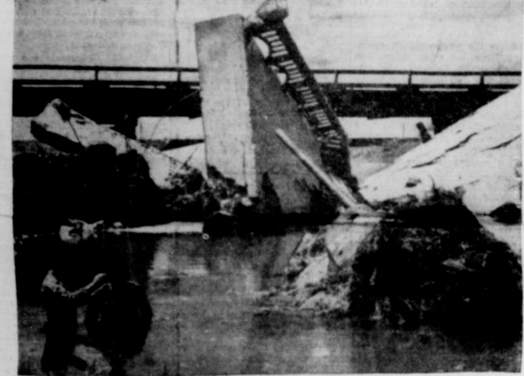
FAITH ON THE BATTLEFIELD—Lt. Kenneth L. Oden of Chicago, Ill., right, is baptized by Capt. Arthur E. K. Brenner, Chaplain, of Bennington, Vt., in the muddy waters of the Chinwihan River in Korea. The devastated bridge in background and the abandoned Russian-made T-34 tank at right testify to the savage fighting that raged in this area previously. (N.S. Air Force photo from Acme).
